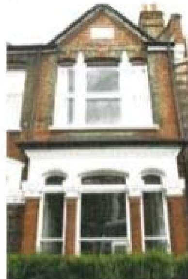
Main picture: the light well brightens the heart of the house. From left: the exterior betrays little of its interior remodelling; the finished office. Top right: storage under the eaves
